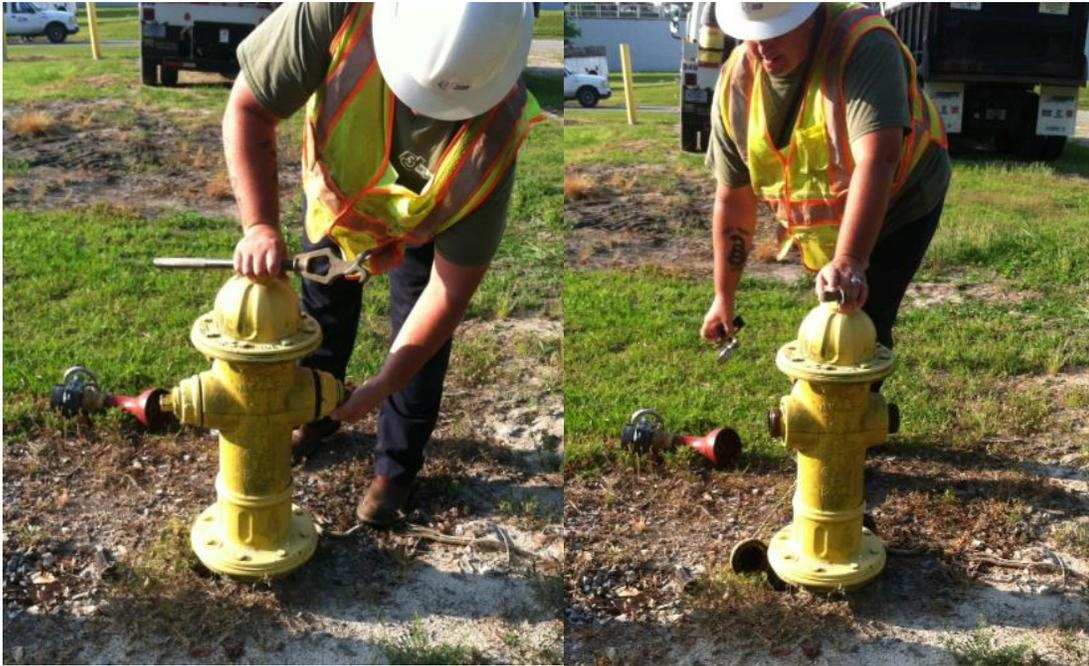
6. Install static gauge on one side and hydrant test valve in the open position with diffuser on other side.
