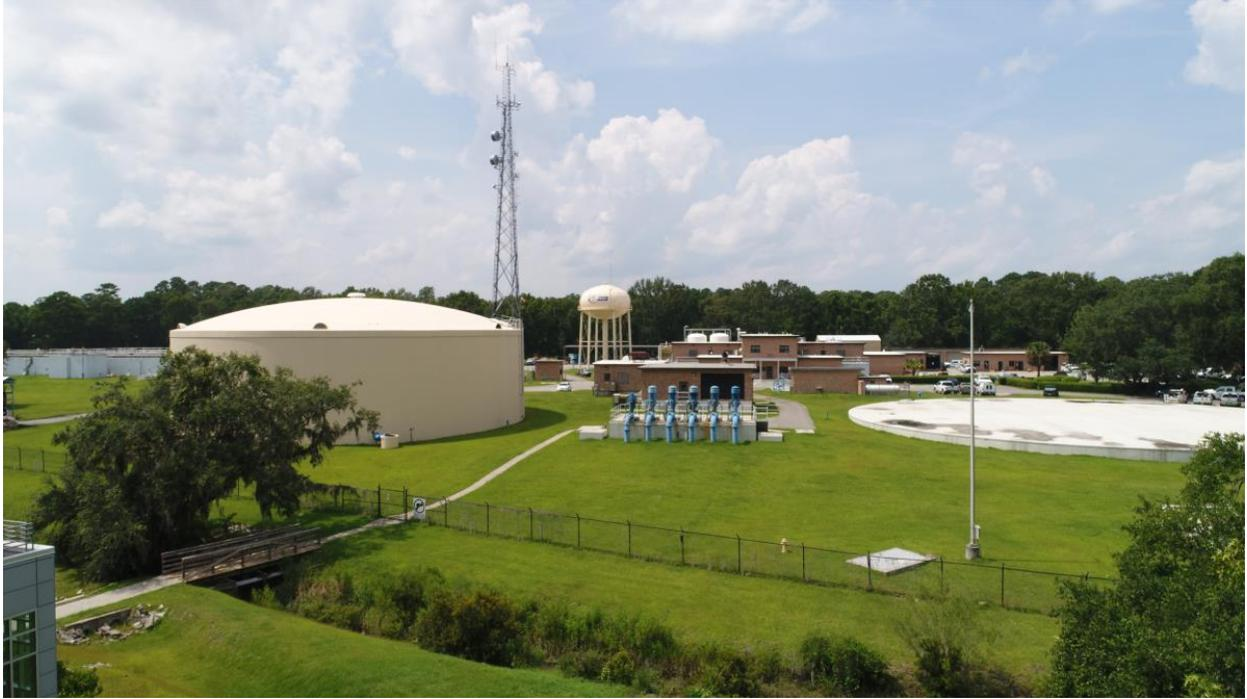
The Chelsea Water Treatment Plant has a 1.5 million gallon clearwell (right) and 3.0 million gallon clearwell (left) which provide contact time for the disinfection process to inactivate viruses and bacteria.
